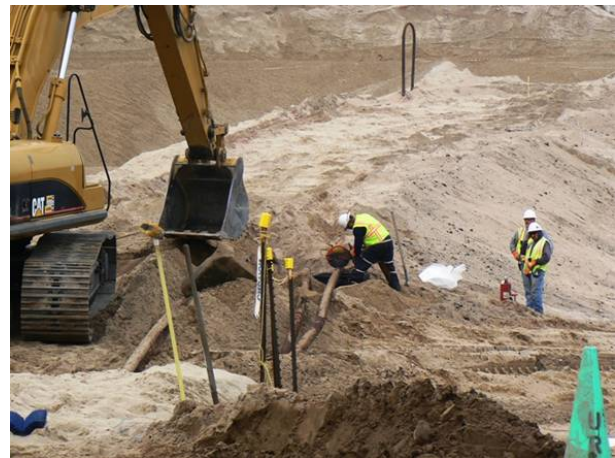
B5A: hot-tapping pipelines before their removal.
