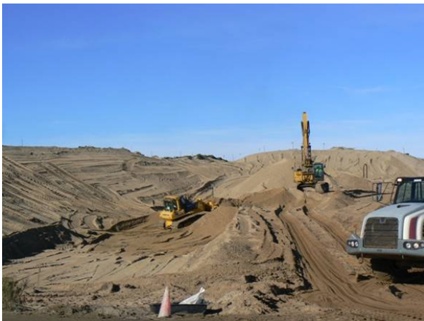
B5A excavation of clean overburden, late December
