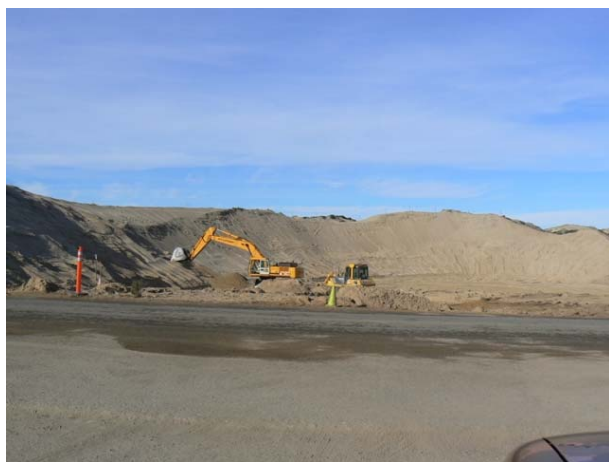
B5A excavation of clean overburden, mid January.
