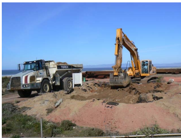
B3A removal of concrete basin.
