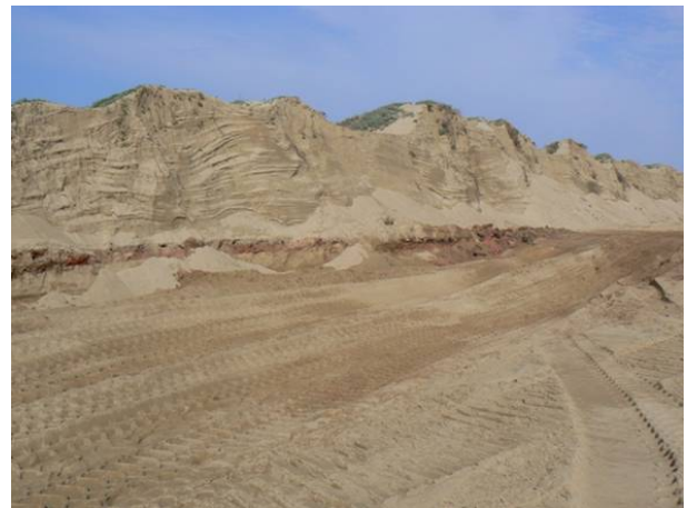
A Road removal; note layer of red rock and road base that will remain in place to preserve functioning foredune habitat above.
