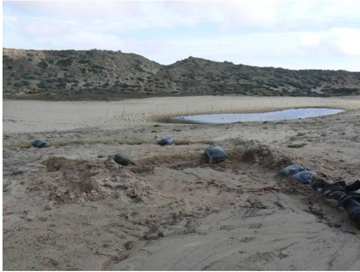
N12 Created wetland: SWPPE repairs (note erosion features) were required at this and several areas on the site during the last storms.
