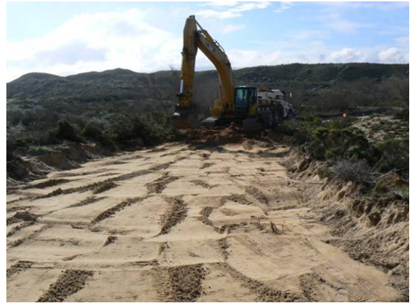
Q5 access road removal.
