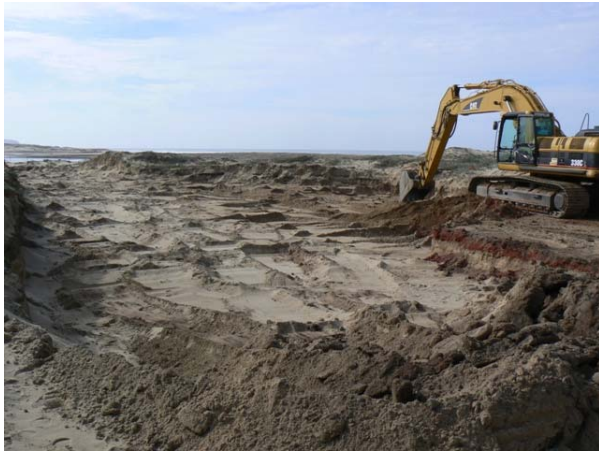
A Road removal.
