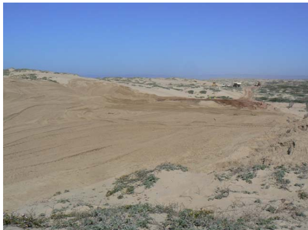
A Road backfilled and re-contoured.
