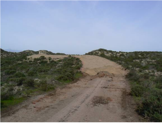
F11 Pad and access road removal.
