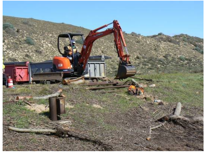
M12 Pipeline removal.
