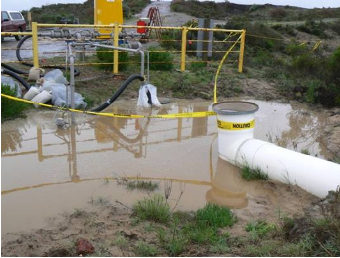
TB9 Stockpile Site: contaminated storm-water runoff overflowed containment.
