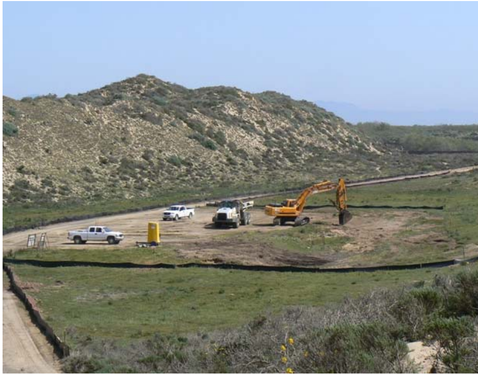
M12 Vegetation removal in preparation for sheetpile installation.
