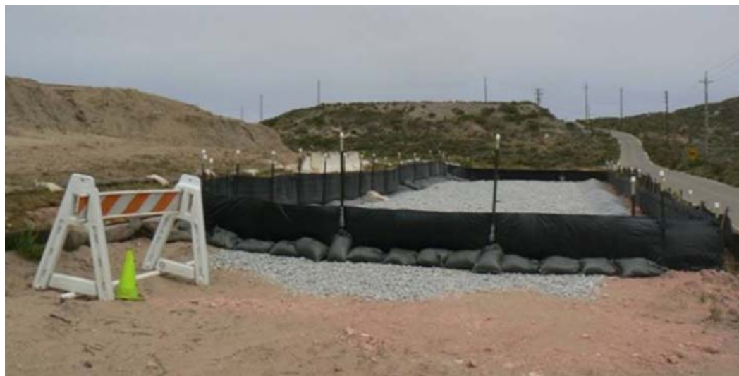
The finished Decon Pad outside the TB9 Stockpile Site.
