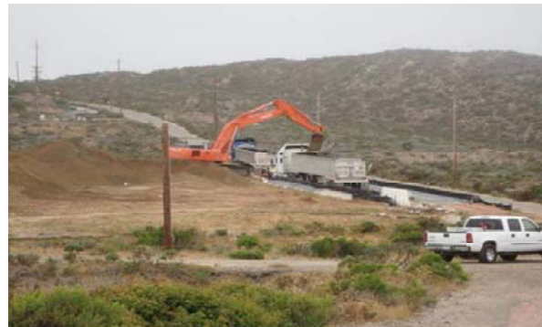
Loading haul trucks at the TB9 Stockpile Site.
