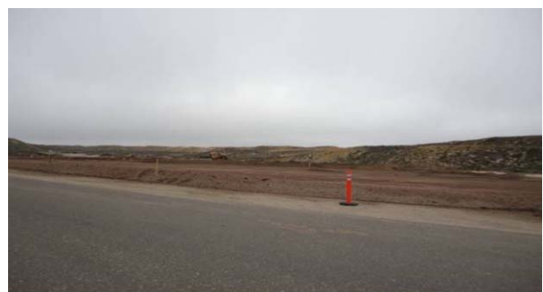
Constructing the new M3 Stockpile site and Loading Zone.
