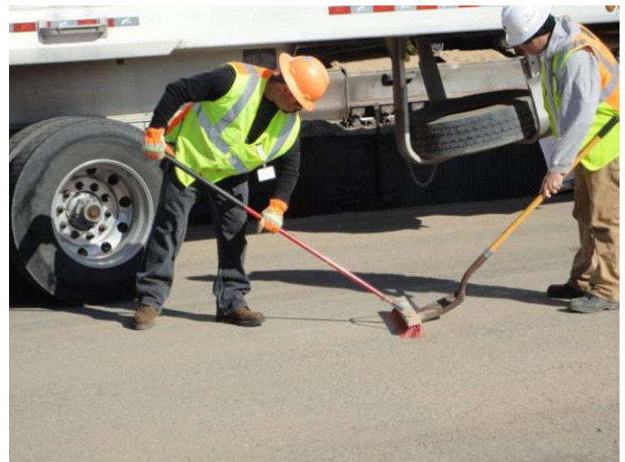
Decontamination cleaning of spilled material at the B5A Site.
