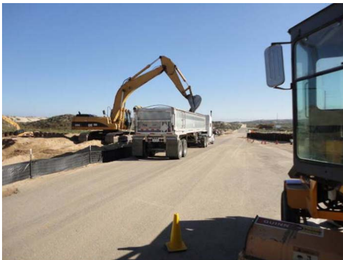
Direct loading end-dump (on-road) haul trucks at the B5A Excavation Site.
